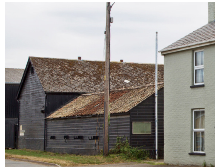
Figure 35: contrasts in the streetscape a. Boxworth End: agricultural buildings in continuous timber weatherboarding with black tar finish.
