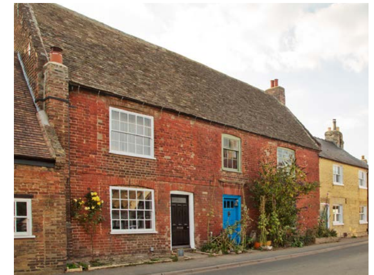
b. High Street: landmark building in red brick at numbers 10-12. The elevation terminates the view from the historic Market Street.
