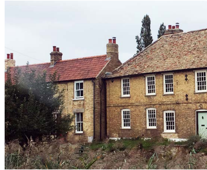
Figure 34: historic palette a. Swan Pond: Buff brick with painted wood windows, clay or pantile roofs.
