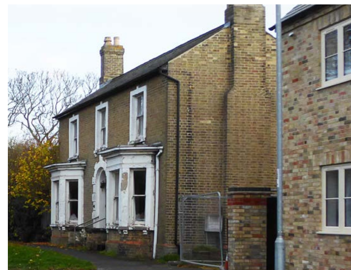
Figure 36: local accents a. Market Street: white render and paint to windows and projecting bays within a unified brick volume.
