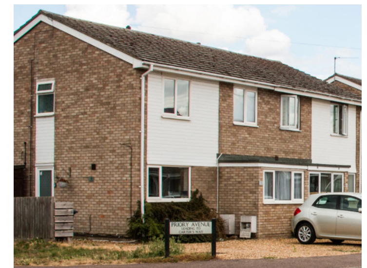
b. Priory Avenue: panels of white painted timber boarding are subservient to the full height brickwork, which turns the corner.
