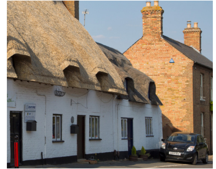
b. High Street: unified brick walls, either limewashed or exposed. Thatched roofs found on a few of the oldest houses.
